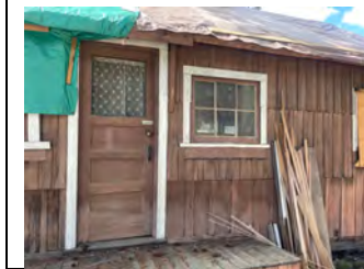
28x14' hut modified as shed. 6-pane sliding windows. Original style roofing & shiplap siding exposed (2nd Ave.)
