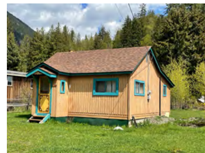
20x14' cabin with lean-to & porch (Kildare St.)
