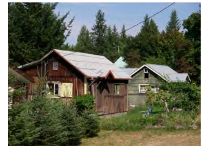
20x14' cabins with half-pitch roofs and lean-to additions in 2006, since updated (Union St.)
