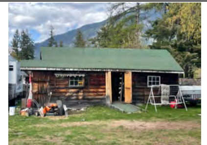
28x14' hut modified as shed. 6-pane sliding windows. Original style roofing & shiplap siding exposed (2nd Ave.)
